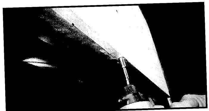
Figure 4. Remove Screw from Top of Appliance Opening
