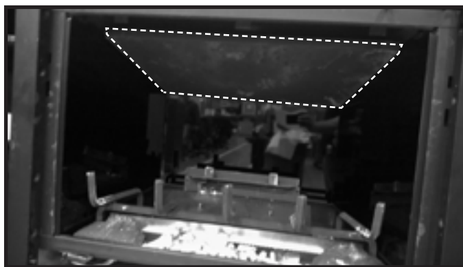
Figure 11.5 Install Top Refractory Panel
