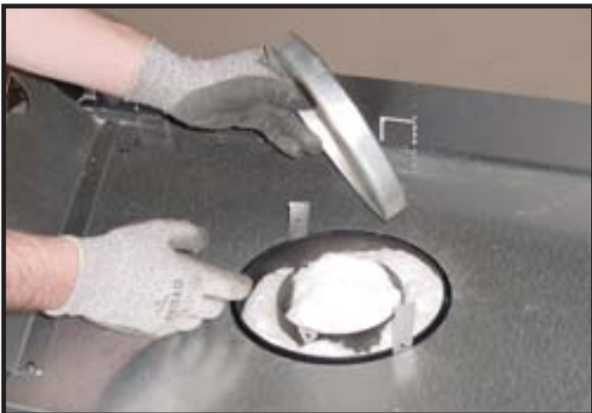
Figure 6.3 (Generic Appliance Shown) Remove the seal cap.
