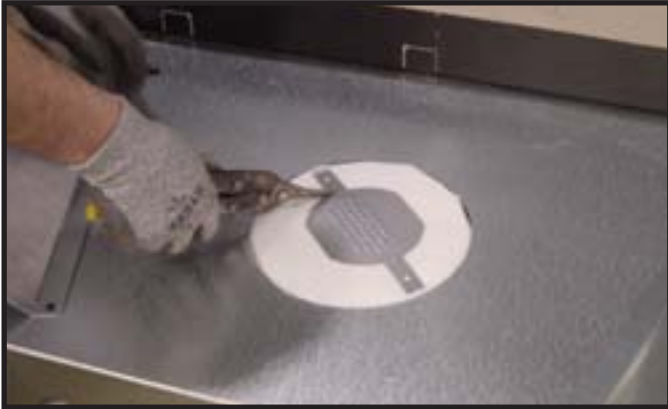
Figure 6.1 (Generic Appliance Shown) Cut the seal strap across the rectangles next to the disk. For rear vent, skip this step.
