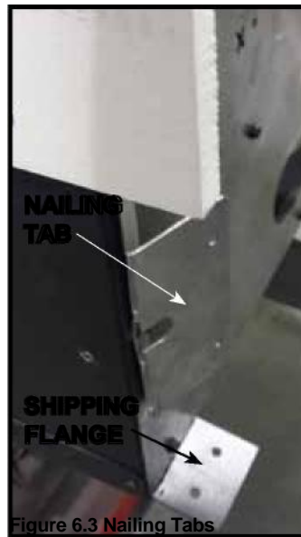
Figure 6.3 Nailing Tabs Shipping Position
