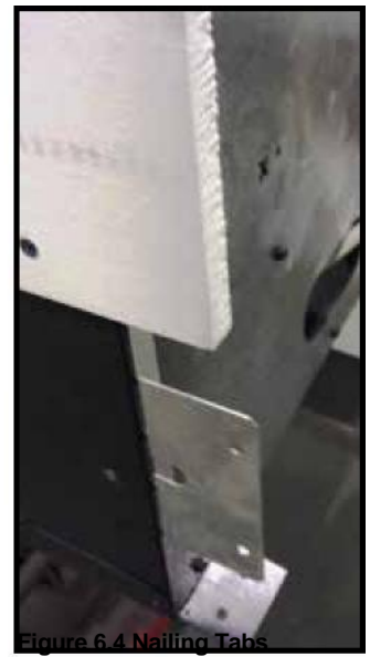
Figure 6.4 Nailing Tabs Installation Position
