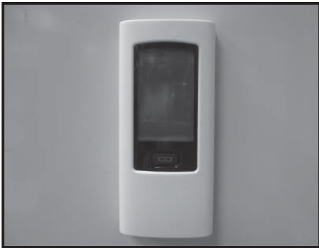
Figure 43. Mounting Remote Control Housing
