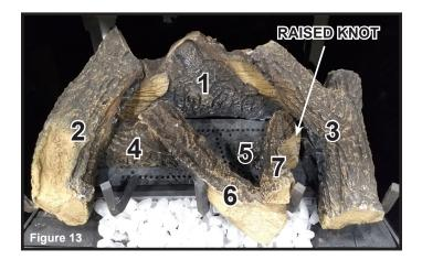
Log #7 (SRV2165-707): Place back (unnotched) end of Log #7 on the flat area on the top of Log #5. Log #7 must be pulled tight to the locating notch. Pivot the front (notched) end of Log #7 to the right until the notch of Log #7 contacts the grate tine located 4th from the left as shown in Figure 13.
